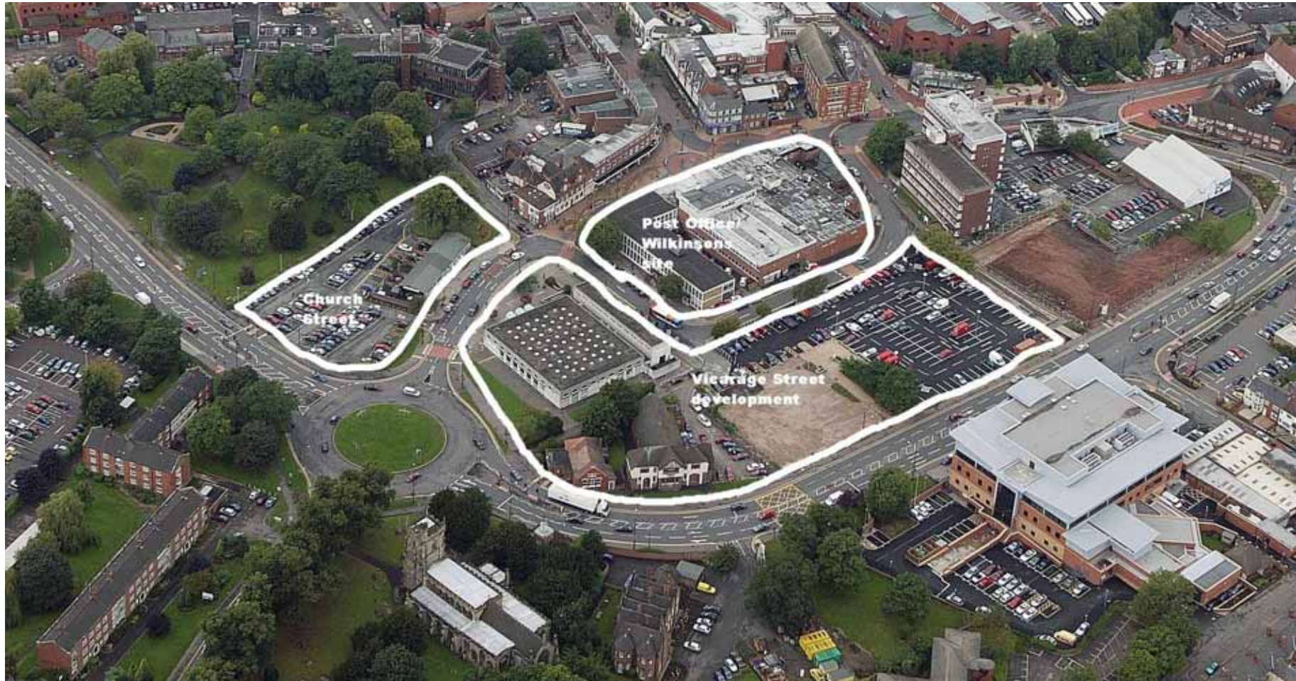
Arial Picture of Vicarage Street site
